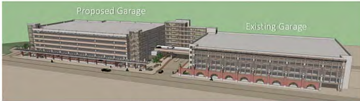
Bird's eye view of Parking Complex
