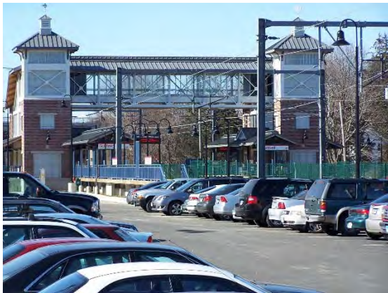
Guilford Shore Line East Station provides for “up and over” access, allowing service on both tracks and parking on both sides of the railroad.
