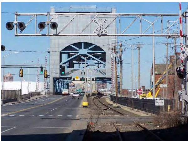
Rail Service across New Haven Harbor has been restored on the Tomlinson Bridge
