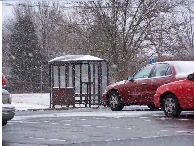
Park and Ride Lots reduce single occupant vehicle usage, reduce highway congestion and, when suitably located, provide intermodal connections.
