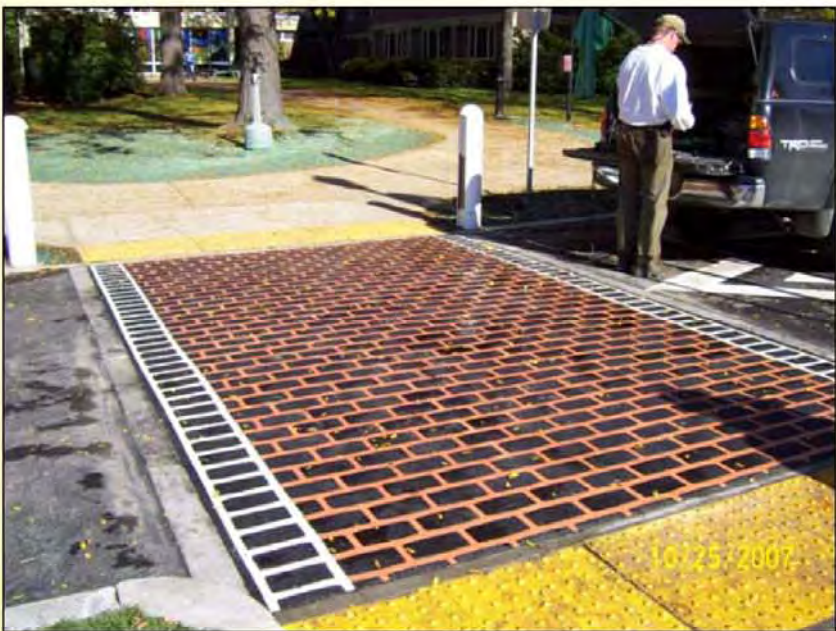
Crosswalk with thermoplastic markings - Main Street in Keene NH (Clough Harbour & Associates)
