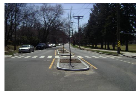
Example of a raised island, West Hartford, CT
