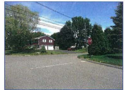
REMOVE VEGETATION IMPROVE SIGHT DISTANCE ALLEN AVE. AT EDGEMARK ACRES LOOKING EAST
