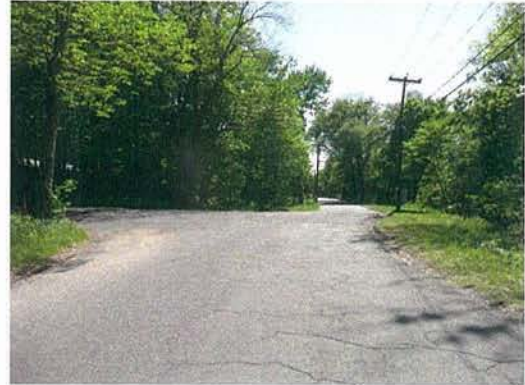
Vegetation obstructs intersection sight distance looking southwest on Allen Avenue
