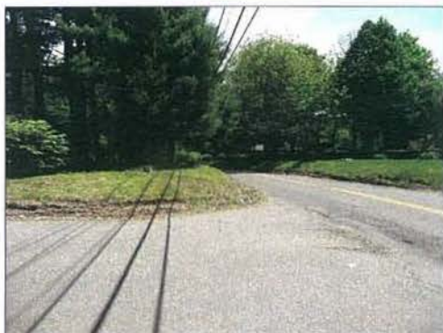
REGRADE SLOPE TO IMPROVE SIGHT DISTANCE ALLEN AVE. AT GOODSPEED AVE. LOOKING EAST
