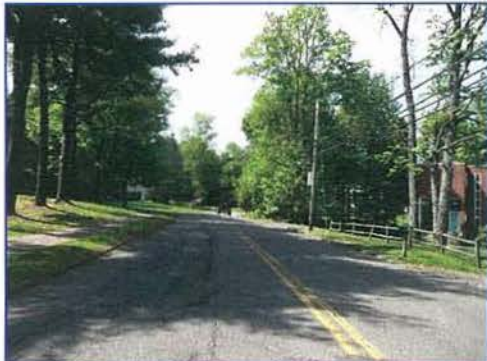
RECONSTRUCT ROADWAY FOR PAVEMENT REHABILITATION ALLEN AVE. EAST OF COE AVE. LOOKING WEST
