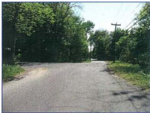
REMOVE VEGETATION TO IMPROVE SIGHT DISTANCE ALLEN AVE. AT FINCH AVE. LOOKING SOUTH
