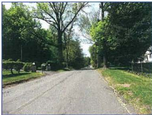
RECONSTRUCT ROADWAY FOR PAVEMENT REHABILITATION ALLEN AVE. AT SPRING GLEN DR. LOOKING WEST
