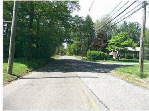
Shrub obstructed intersection sight distance looking southwest at Spring Glen Drive
