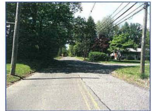
REMOVE VEGETATION TO IMPROVE SIGHT DISTANCE ALLEN AVE. AT SPRING GLEN DR. LOOKING WEST
