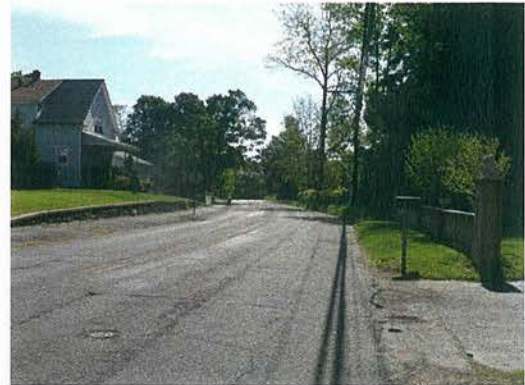
Horizontal curve on Johnson Avenue east of Fiesta Heights (East)
