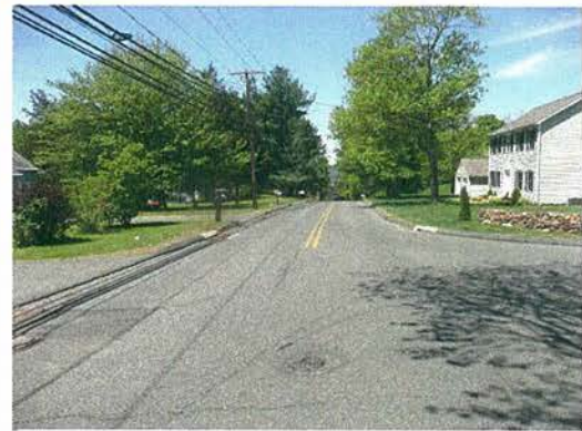
Johnson Avenue narrows at Gwen Road intersection
