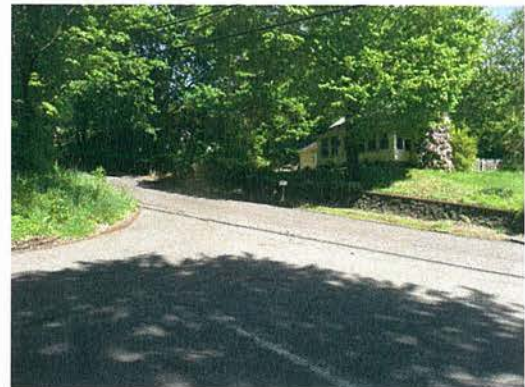
Steep vegetated slope inhibits intersection sight distance on Goodspeed Avenue looking west
