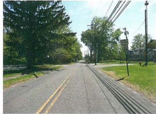
Narrow roadway on Johnson Avenue looking east towards Sperry Lane
