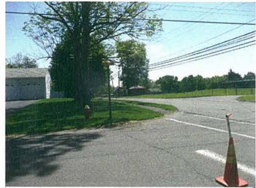
Vegetation between Alanby Lane and Sperry Drive on Johnson Avenue inhibits intersection sight distance looking left from Alanby Drive
