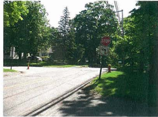
Vertical crest curve inhibits sight distance on Johnson Avenue at Fiesta Heights (West)
