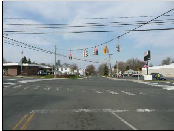
(right) NB E. Main and Gravel
