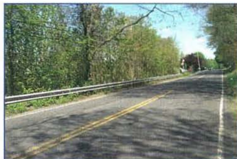
POTENTIALLY WIDEN ROADWAY TO 26' PRESTON AVE. AT PATTON DR. LOOKING EAST
