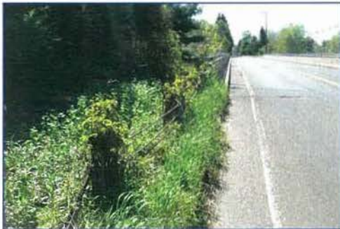
REPLACE OBSOLETE WIRE ROPE RAIL PRESTON AVE. OVER ROUTE 66
