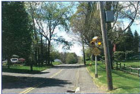
RECONSTRUCT ROADWAY TO IMPROVE SIGHT DISTANCE BALDWIN AVE. AT MATTABASSET DR. LOOKING WEST
