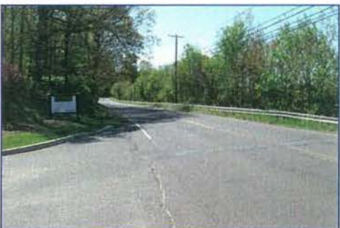
REMOVE VEGETATION TO IMPROVE SIGHT DISTANCE PRESTON AVE. AT PATTON DR. LOOKING SOUTH
