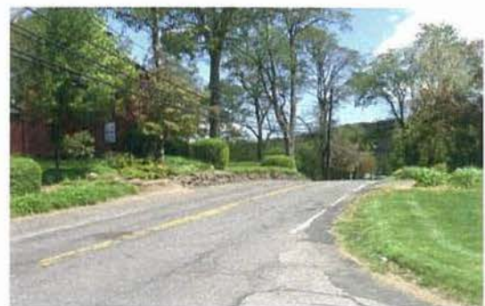
Limited intersection sight distance looking east from Winding Brook Drive
