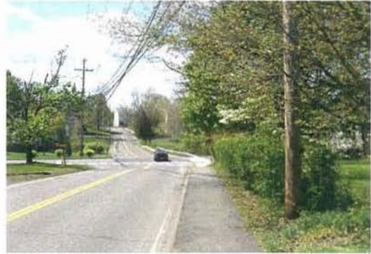
Sight obstruction on westbound approach to Bee Street / Baldwin Avenue intersection
