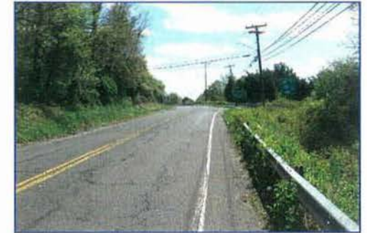
REGRADE SLOPE FOR POLICE ACADEMY DRIVE PRESTON AVENUE LOOKING EAST TOWARDS ROUTE 66
