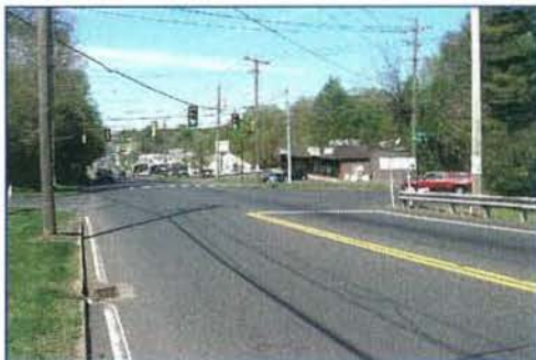
FULL SIGNAL REPLACEMENT EAST MAIN ST. AT PRESTON AVE.
