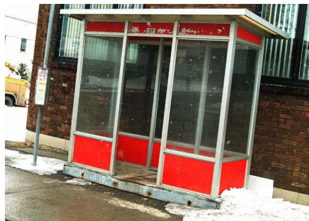
Transit Shelters provide necessary refuge from the elements to users that are more susceptible to harsh weather conditions.
