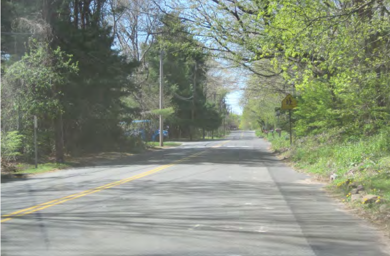
Southbound view near Jackson Road. Crosswalk in distance is barely visible, warning signage is partially obscured by vegetation.
