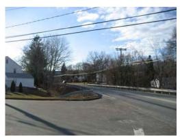
Chestnut Street – Visibility from the northbound approach of Chestnut Street at North Main Street is poor due to grade issues, a curve in North Main Street and an awkward horizontal alignment at the intersection. High prevailing travel speeds in this area have raised concerns over accident potential. Realigning the intersection would not be cost effective due to engineering constraints and right-of-way limits. Volumes at this intersection are not expected to meet signal
