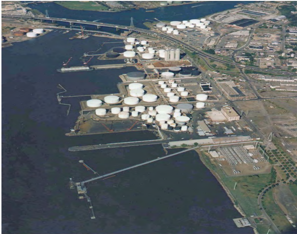
Port of New Haven (Courtesy CDOT)
