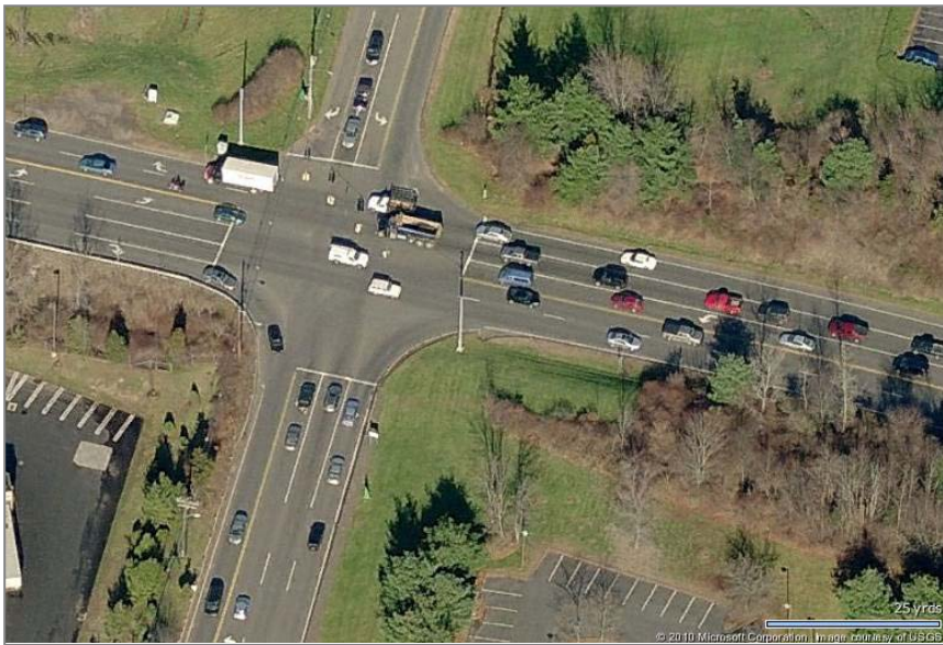
Route 68 at North Main Street Extension Bird's Eye View Looking North
