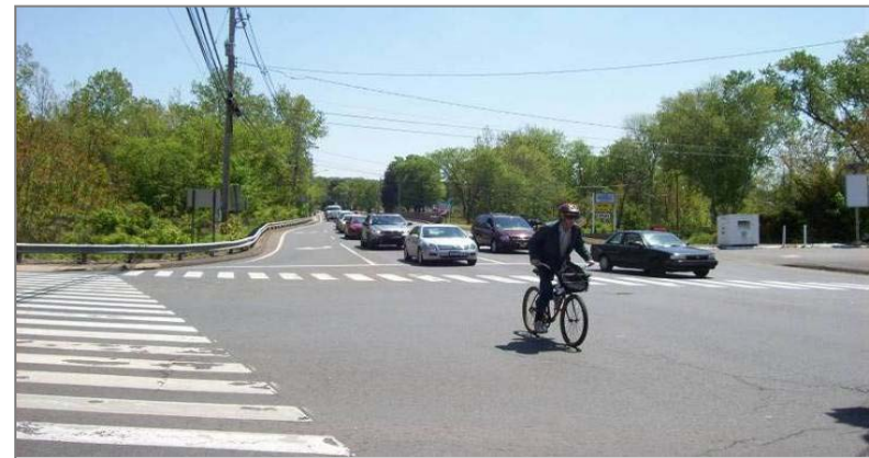
Westbound Traffic on Route 68
