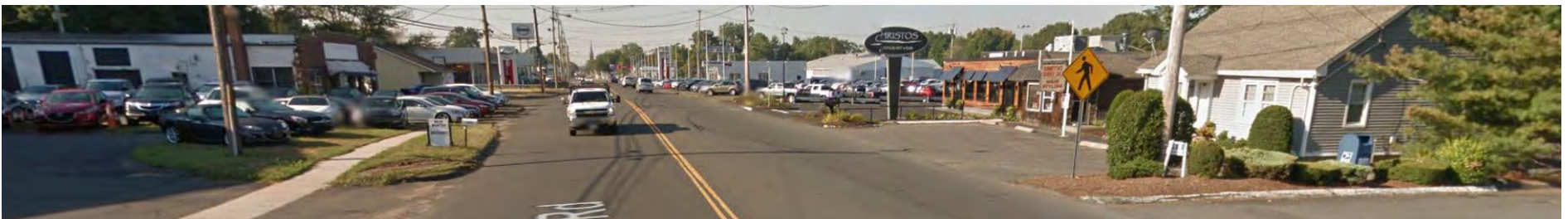
No crosswalk at marked pedestrian crossing on South / North Colony Road (Image credit: Google Street View)
