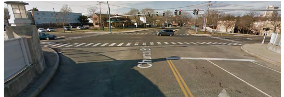
Intersection of Union Avenue and Church Street (Image credit: Google Street View)
