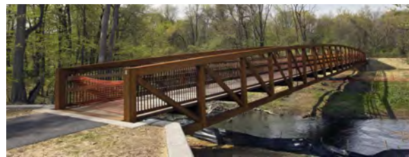
Pedestrian bridge for Quinnipiac River Linear Trail in Wallingford (Image credit: My Record Journal)
