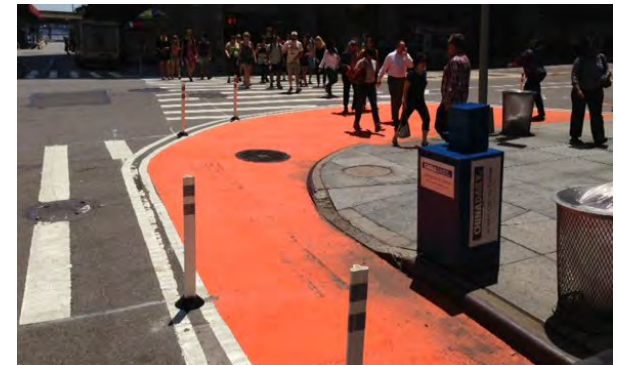
Curb bump-outs can be painted as a low-cost, temporary installation during a trial period along a roadway (Image credit: Clarence Eckerson Jr. via StreetsBlogSF)
