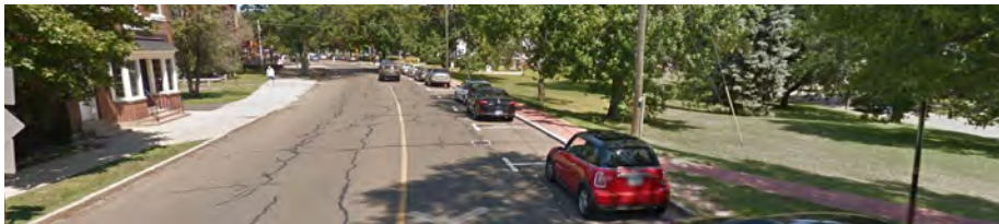
Cross-section along Route 146 where pedestrian crashes have occurred (Image credit: Google Street View)
