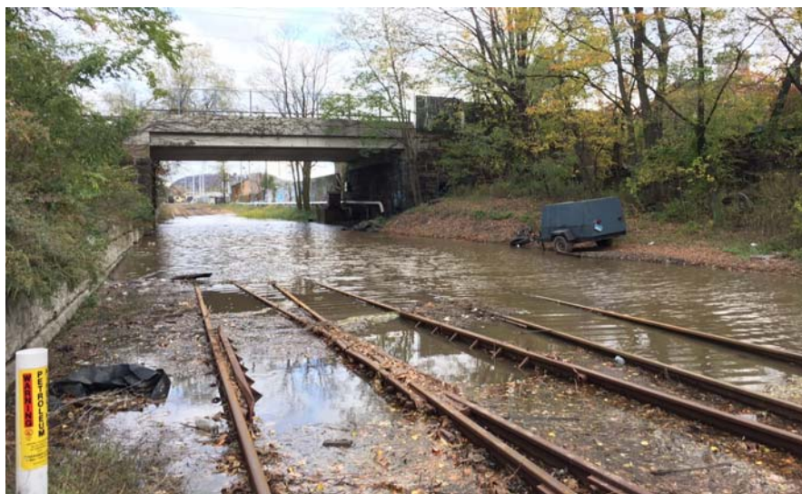
Figure 2-15. Flooding under Chapel Street
