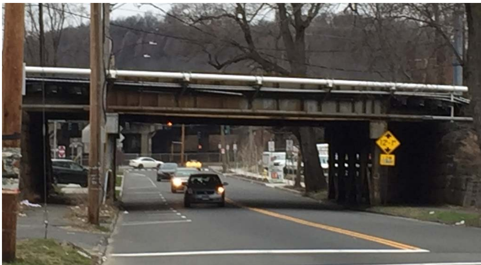
Figure 2-13. James Street Overpass
