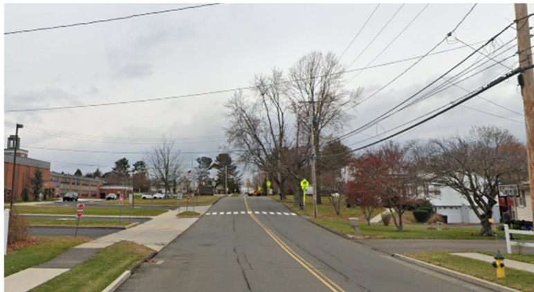
Morgan Lane near Bailey Middle School- sidewalk ends without connecting to the marked crosswalk (Source: Google Maps)
