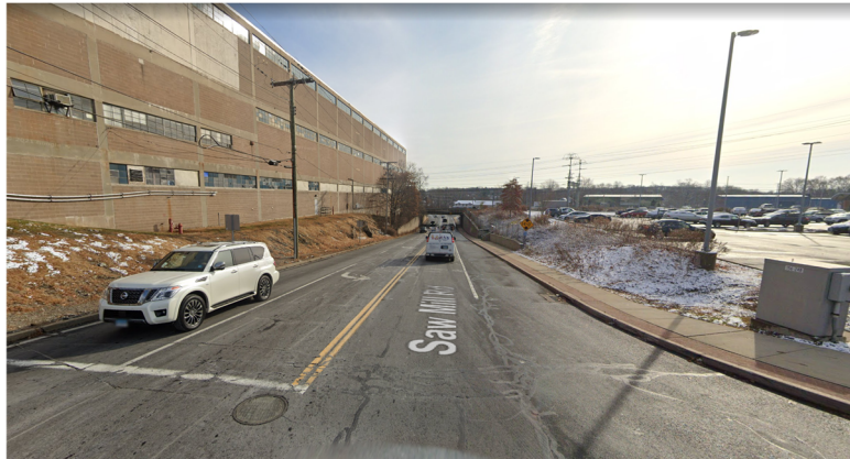
Saw Mill Road south of Railroad Avenue- no sidewalk is provided along the East side of the roadway (Source: Google Maps)
