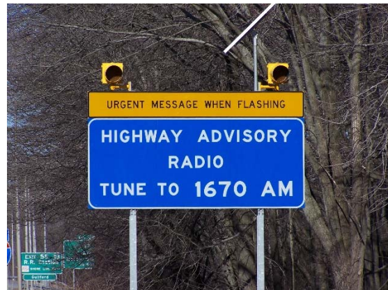
Variable Message Signs and Highway Advisory Radio provide important travel information for reducing congestion and travel delays due to highway incidents.
