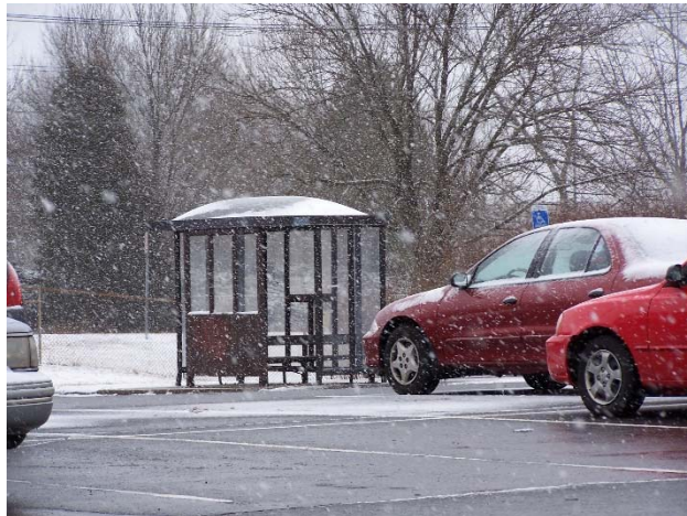
Park and Ride Lots reduce single occupant vehicle usage, reduce highway congestion, and when suitably located, provide intermodal connections.
