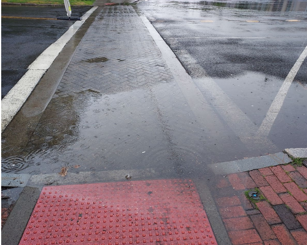
Figure 9 Flooded Curb Ramp – Whitfield Street at Boston Street
