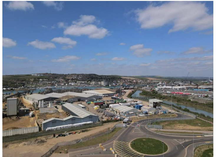
Figure 3: Port of New Haven Facilities
