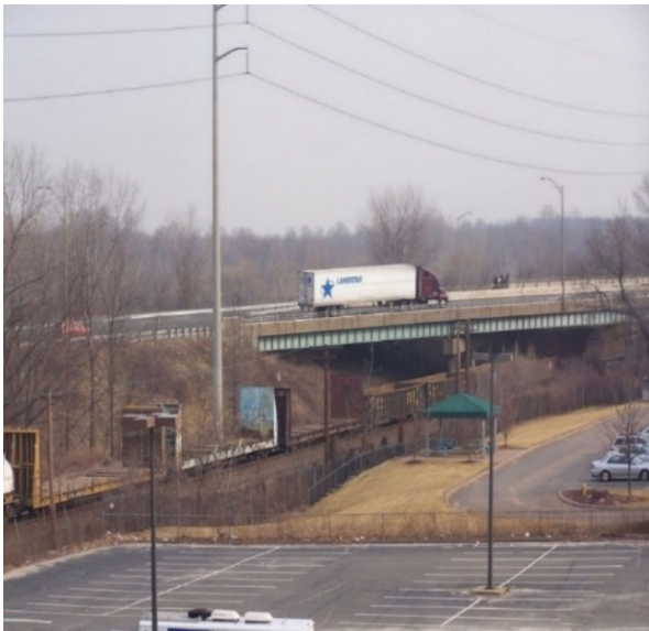
Freight movement is a critical component of the regional transportation system. Increased rail utilization will remove trucks from the Region's highways and help reduce highway congestion
