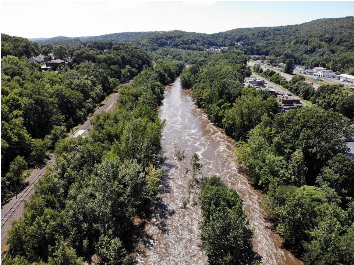
Photo: Naugatuck and Housatonic Rivers following the remnants of Hurricane Ida
