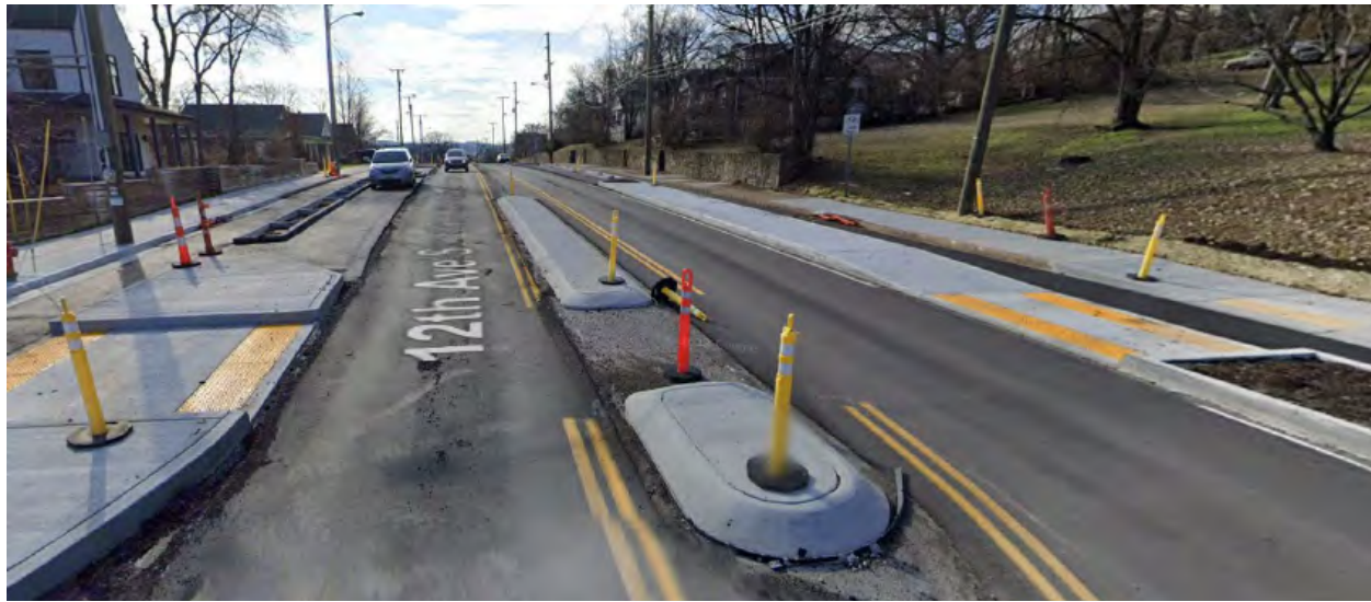
Figure 4.18 Pedestrian Refuge Island – Nashville, TN
