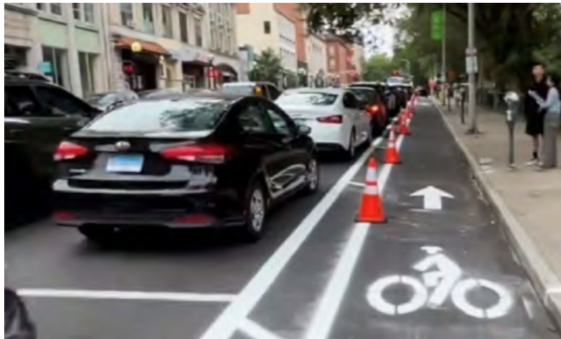
Figure 2.10 Parking-Protected Bike Lane on Chapel Street between Temple Street and College Street
