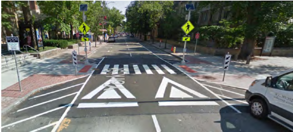
Figure 2.9 Mid-Block Raised Crosswalk on York Street
