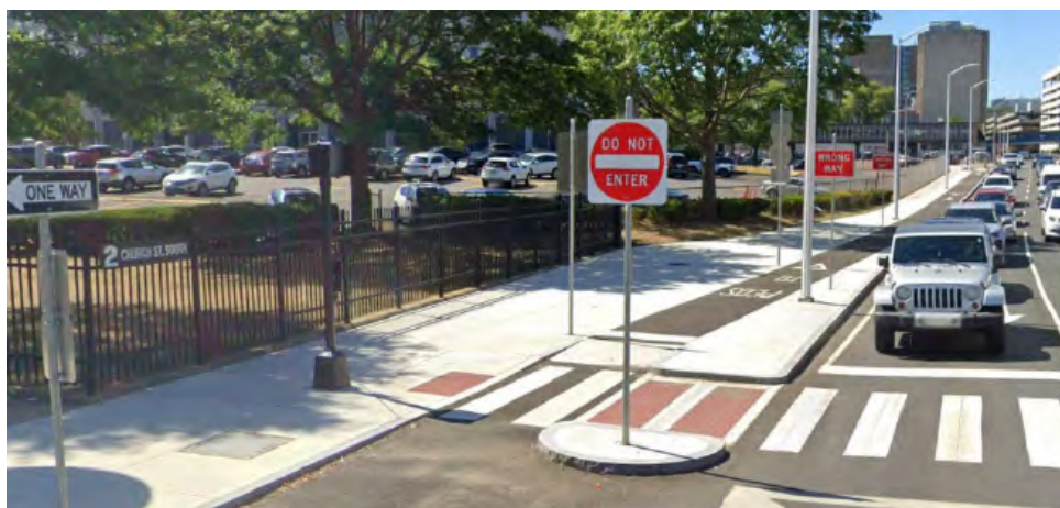
Figure 2.11 Sidewalk-level Bike Lane South Frontage Road Downtown Crossing
