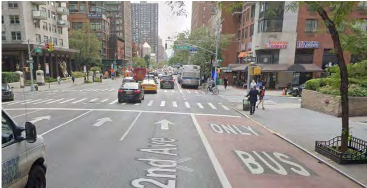
Figure 4.16 Curbside-Running Bus-Only Lane – New York, NY
