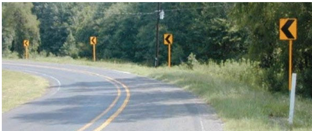
Figure 18 Chevron Alignment Signage with Retroreflective Sheeting (Source: FHWA)
