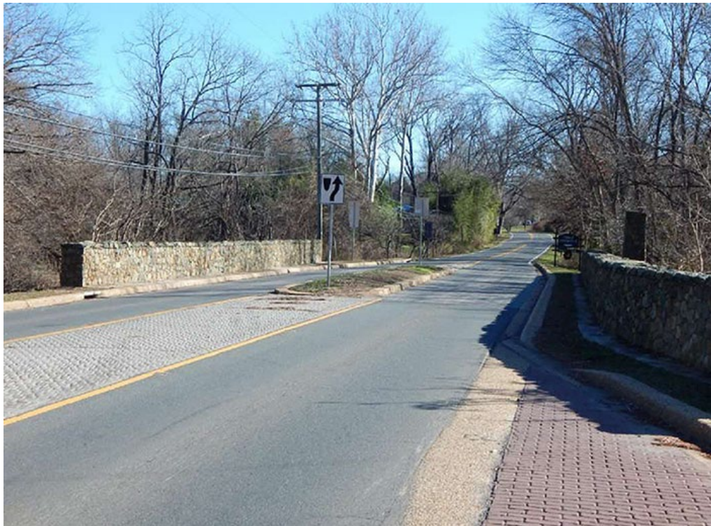
Figure 25 Raised Median Island (Source: FHWA)
