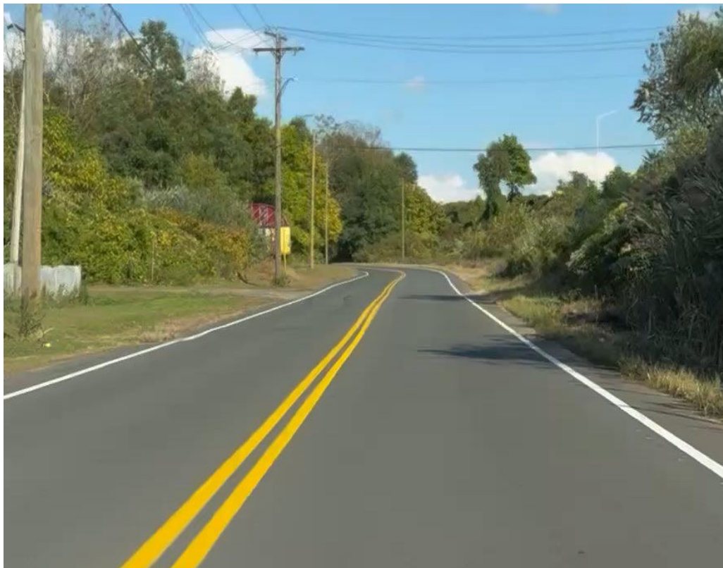
Figure 3 Valley Service Road
