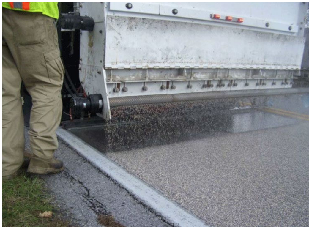
Figure 20 High Friction Surface Treatment Application (Source: FHWA)
