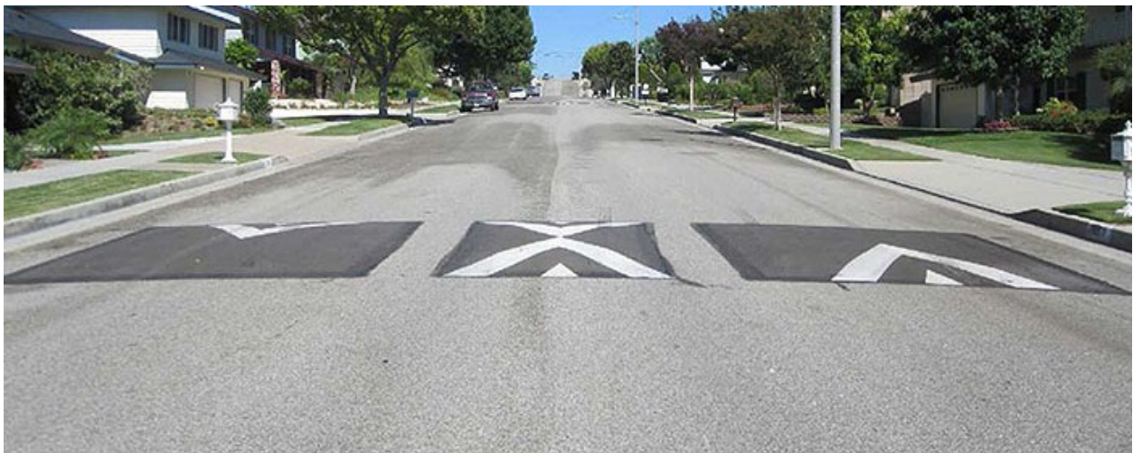
Figure 23 Speed Cushion (Source: FHWA)
