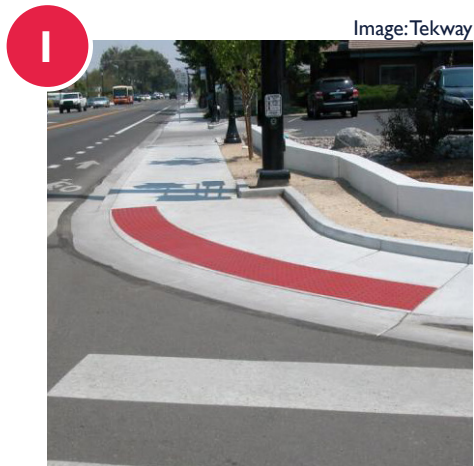
ADA-COMPLIANT CURB RAMPS
