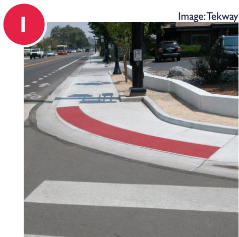
ADA-COMPLIANT CURB RAMPS
