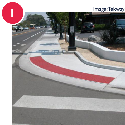
ADA-COMPLIANT CURB RAMPS
