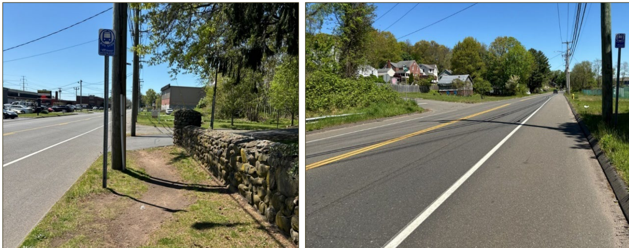
Figure 8 State Street – Typical Bus Stop Conditions north of Fernwood Road (left: southbound bus stop at Highvue Manor in the grass buffer area, right: northbound bus stop at Craft Street in the roadway shoulder)
