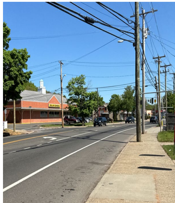
Figure 4 State Street, looking north at Farm Road
