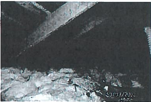
Figure 3. Attic space showing wooden roof shingles.
