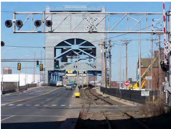
Rail Service across New Haven Harbor has been restored on the Tomlinson Bridge
