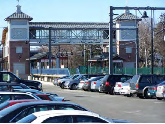
Guilford Shore Line East Station provides for “up and over” access, allowing service on both tracks and parking on both sides of the railroad.
