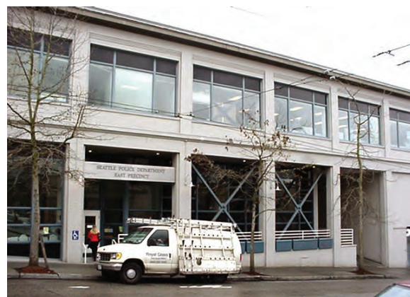
A seismic retrofit of this police station in Seattle, Washington was paid for using capital improvements funds. Structural bracing was added to the building at all levels. The project is highlighted in FEMA's Best Practices Portfolio.
