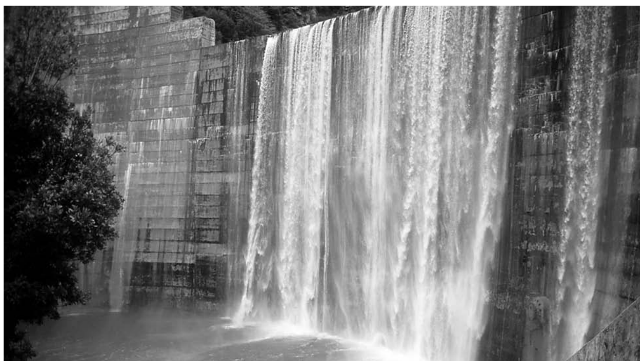
Matilija Dam on the Ventura River in California. Photo credit: Mark Capelli.
