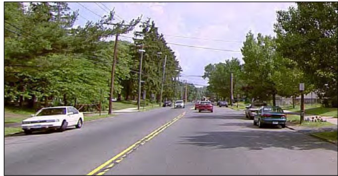
The view along northbound Ella T. Grasso just south of Edgewood Park shows a 48 ft wide roadway with a single centerline stripe and on-street parking that is not defined with pavement markings.
